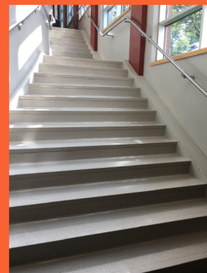
The worn carpeting on the library's main staircase was replaced with heavy-duty rubber stair treads with risers.
